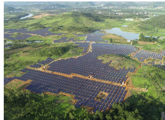
Poverty Alleviation PV Power Station in Jianghua Yao Autonomous County, Hunan Province
